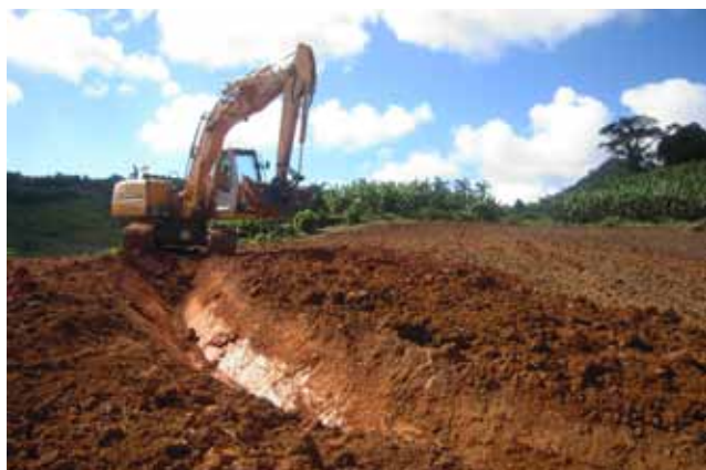
Digging of drainage canals - Photos IT 2
